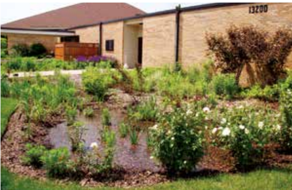
A well-maintained rain garden at Vision of Glory Lutheran Church captures and cleans storm water runoff.
